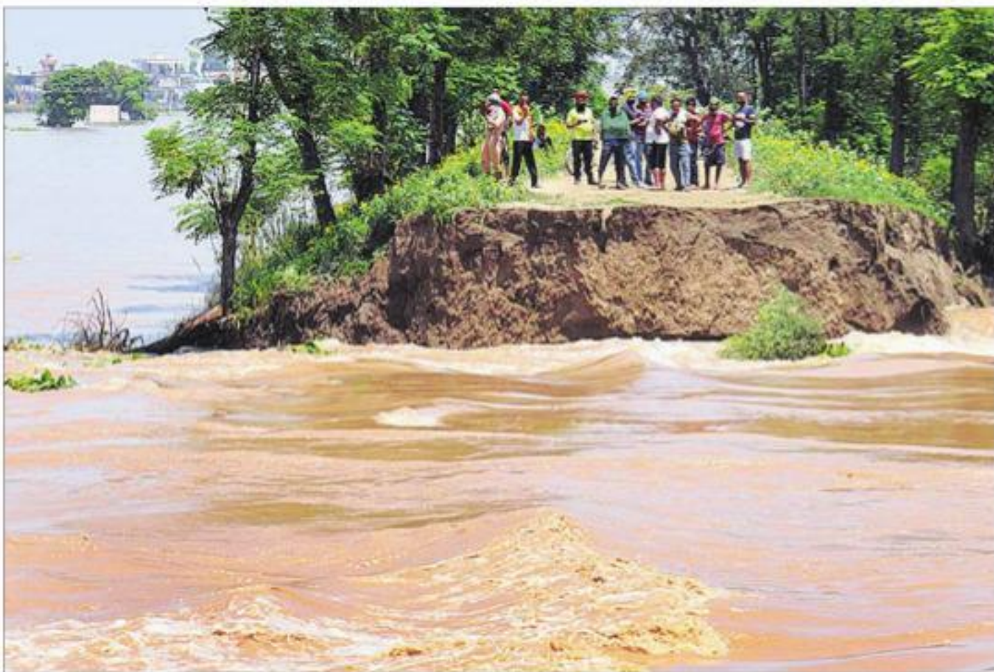
A breach in the Dhussi bundh along the Sutlej in Shahkot. TRIBUNE PHOTO: MALKIAT SINGH
